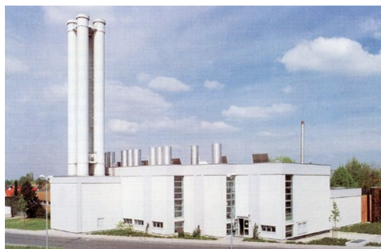
THE ENERGY CENTER provides Mohn Media with electricity, heat and cold.
